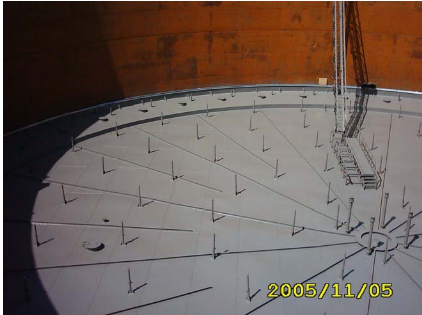
fig. 6 Stiffening of membrane with radial girders, Sudan
