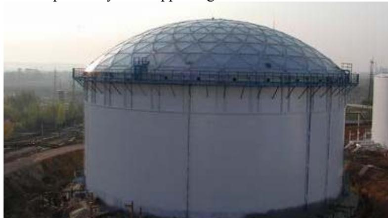
fig. 7 Aluminum dome roof
