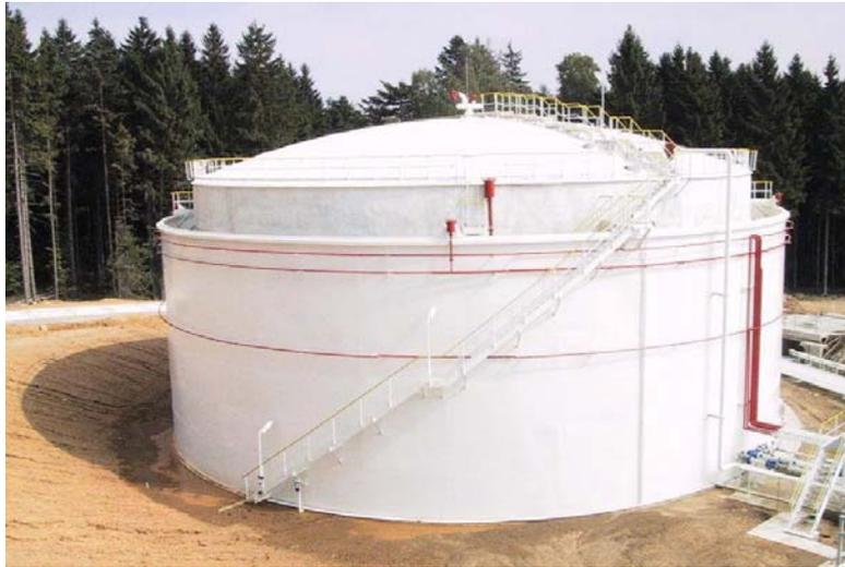
fig. 5 Tanks with double steel shell
