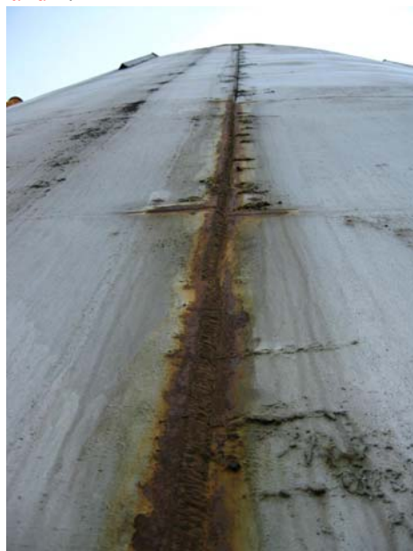
Fig. 2. Vertical welding joint, made on site
