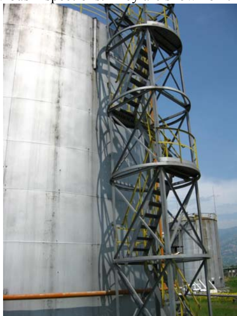
Fig. 1. Steel tank – general view
