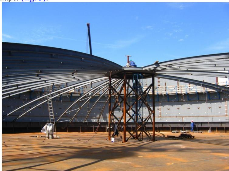
fig. 3 Temporary support for roof assembling
