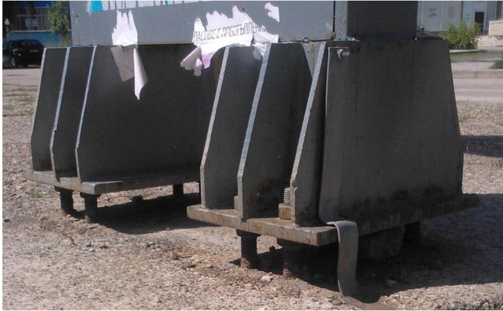
**Fig. 10. Anchor bolts with nuts under the base plate. Execution.**
