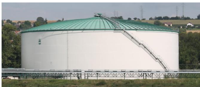
Fig. 1. Aboveground steel tank with V = 70\,000\text{ m}^3 capacity for molasses
