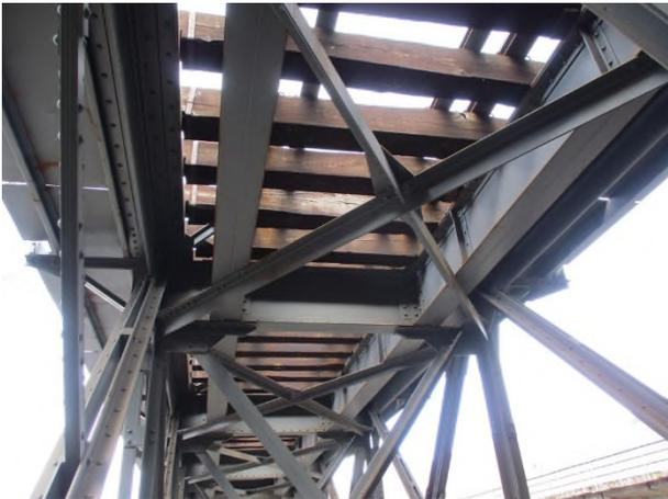
Figure 2. "Open type" deck structure
