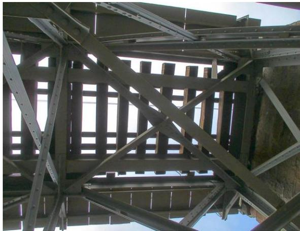
Fig. 2. "Open type" deck structure
