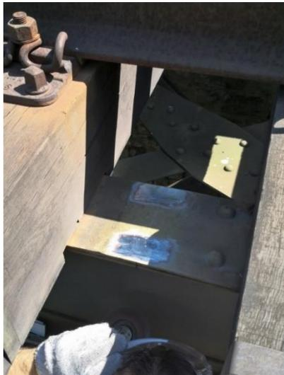
a) cleaning of the flanges of the longitudinal beams
