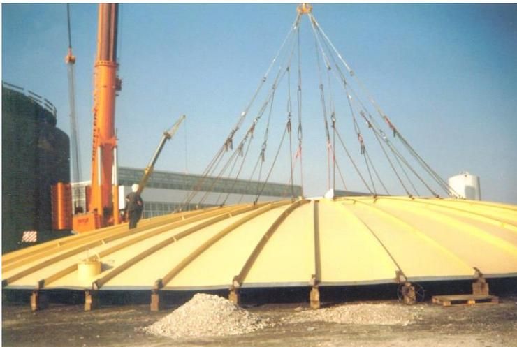
*c) assembling on the ground and lifting as one piece*
